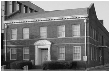
Old OMU Building
